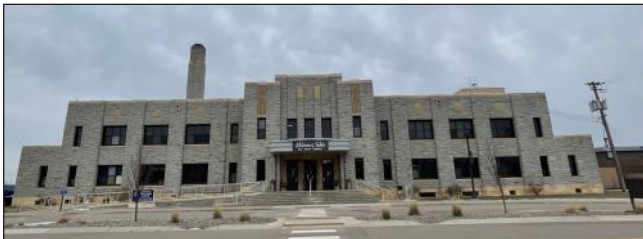
The terminal at Saint Paul's downtown Airport, also known as Holman Field, was erected in 1939. The building is faced with Platteville Limestone.
