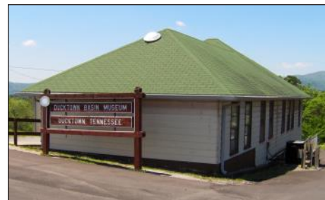
Ducktown Basin Museum, formerly the engineer's office building. Photo by Brian Stansberry, Creative Commons
