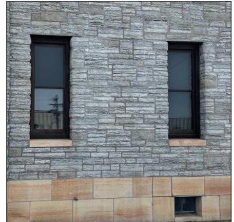
Mankato-Kasota Limestone runs along the base of the building. Irregular-sized blocks of Platteville Limestone face the building's exterior. Note how the stacked stone blocks frame the windows.
