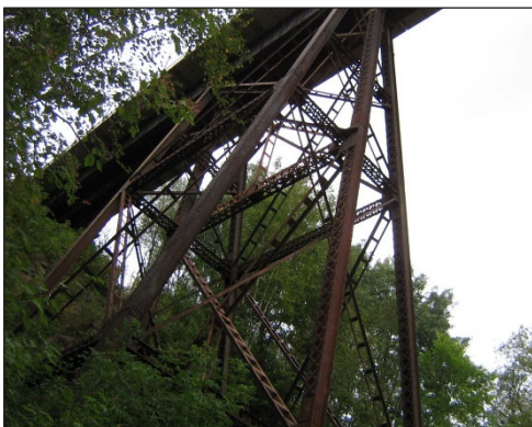
One end of the railroad bridge, photo Mary Helen Inskeep
