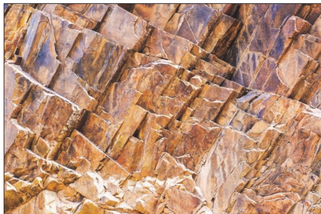
Fractured rocks along Window Trail
