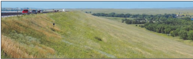
The earthen Kingsley Dam
