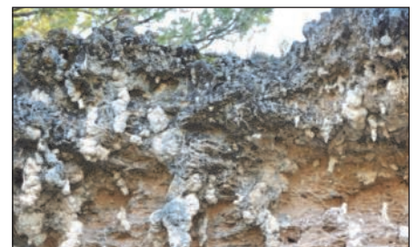
Cavities filled in by more resistant material
